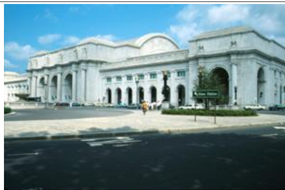
Figure 32 : Washington, Union Station
